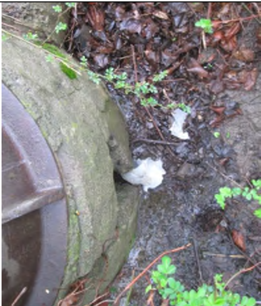
Photo 8: Broken storm drain within wetland (4.21.17)
