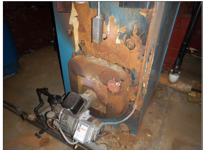
28. Photograph of oil-fired boiler.
