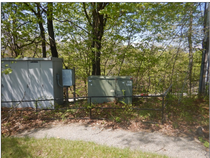
17. Photograph of pad mounted transformer.
