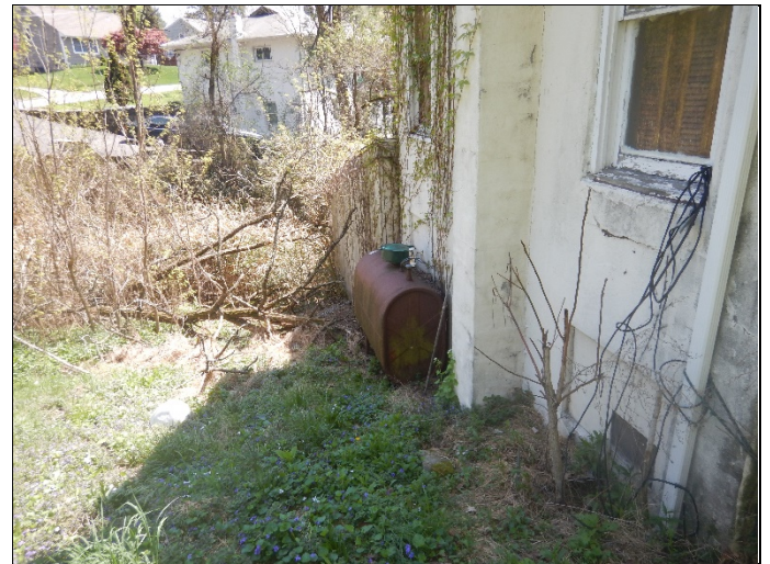
22. Photograph of AST outside maintenance building.
